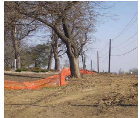
These trees have suffered root damage from compaction and trenching close to their trunks, and will unfortunately decline in the years to come.
